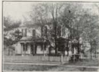
Rev. Molitor Residence
