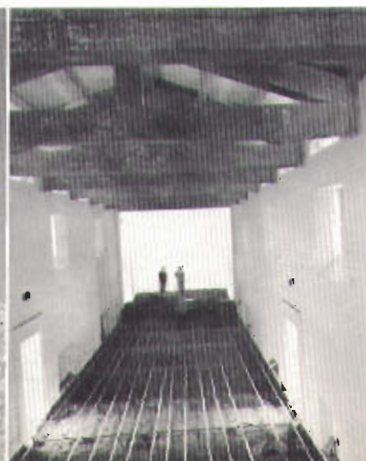
The Vixian Webb Chapel at the Webb School, Claremont, California, radiant heated with NATIONAL PIPE.
