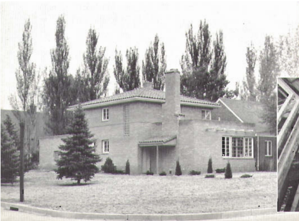
Residence of Elmo Hall, Denver, Colorado. Radiant heating with NATIONAL Steel Pipe installed throughout.
