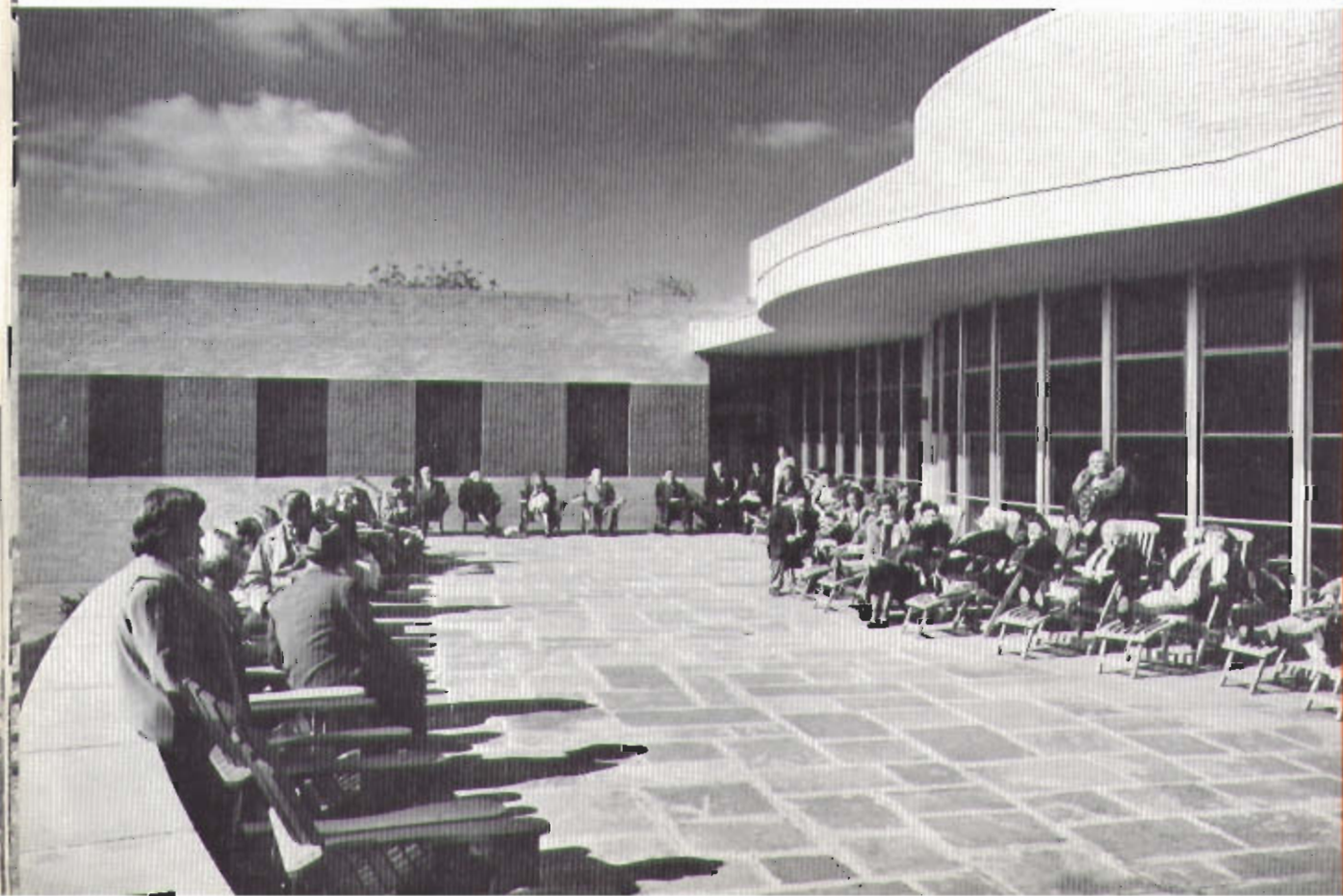
Snow melting coils under this outdoor terrace of Home for Convalescents keep the terrace free of snow and comfortable for longer periods.
