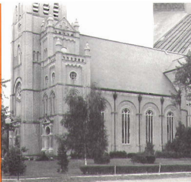
St. John's Church in Delphos, Ohio, is a good example of a hard-to-heat building made comfortable with radiant heating. The auditorium in this beautiful old stone church is 135 feet x 65 feet. The vaulted ceiling is 60 feet high. Here was a natural for radiant heating.
