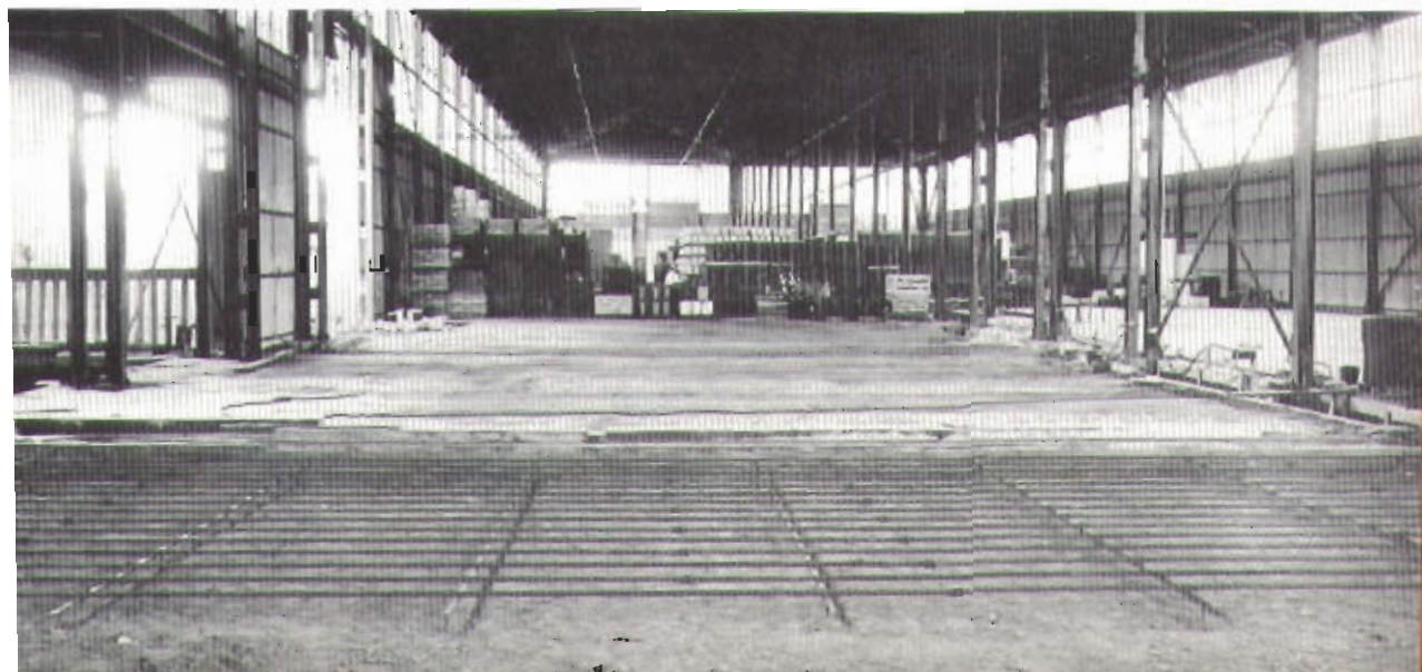
Figure 5. Radiant heating coil is shown embedded in concrete which has been poured on a bed of packed gravel.
