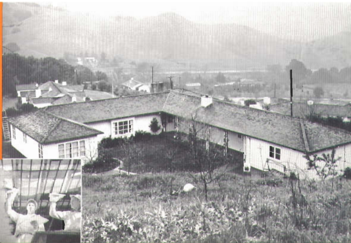
A total of 4000 feet of NATIONAL Steel Pipe was used for the radiant heating system in the residence of Jack Pahl, eastern San Francisco Bay area, California.
