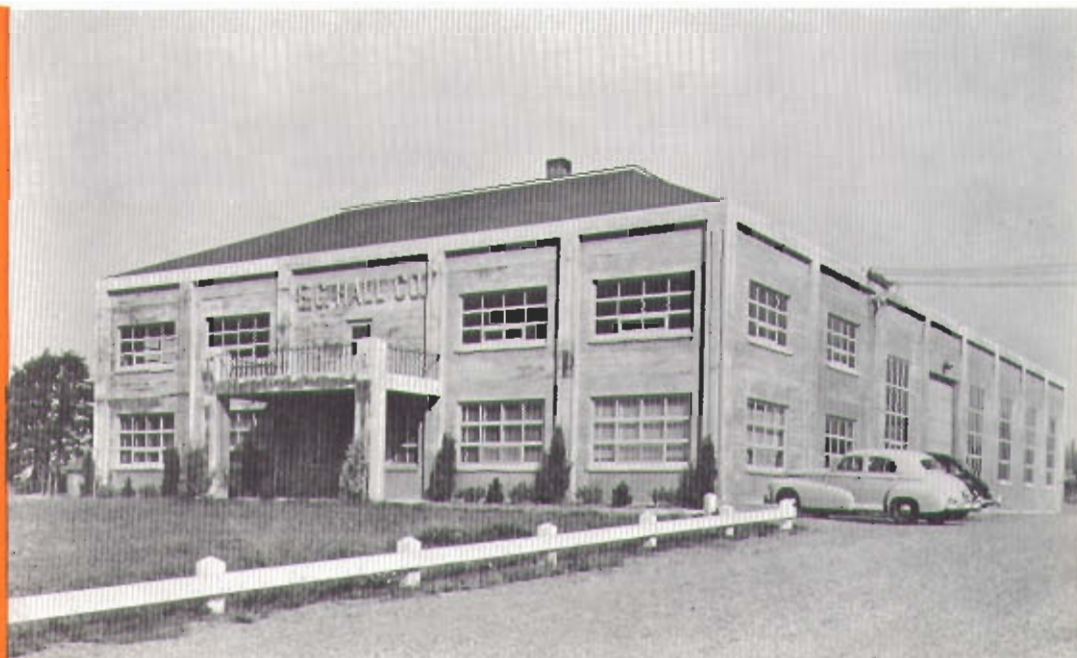
E. C. Hall Company Building at Tigard, Oregon, radiant heated with NATIONAL Steel Pipe.
