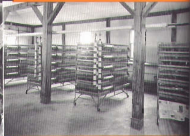
Battery of hoyer trays at Kroeger Turkey Farm. Trays heated by hot water by means of 1/2-inch NATIONAL Steel Pipe coils. The floor panels are 1 1/4-inch NATIONAL Steel Pipe embedded in concrete.
