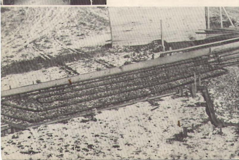
about 80°F. and a water temperature in the coils of about 130°F. This, of course, permits operation at higher water temperatures and higher floor temperatures whenever it is desirable to use air temperatures in the 68-70°F. range.
