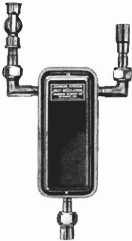
FIG. 22: TYPICAL SINGLE POINT CUMULATOR
