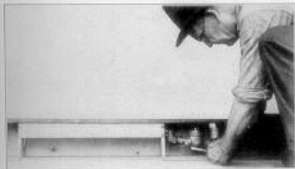
Fig. 38. After taking off the removable baseboard on the concealed installation shown in Fig. 37, the first step toward removing the concealed heater is to disconnect the trap collar and remove the radiator trap. The radiator union elbow in the supply pipe is also disconnected at this time.
