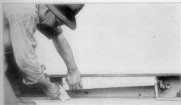
Fig. 39. Next, lift U-bend end of heater as high as it will go and remove leg. This operation shows importance of having clearance between bottom of stack and shoulder on heater, as illustrated in Fig. 28, page 22.
