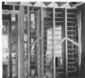
Radiant Heating copper pipes were installed in the dressing-room wall.
