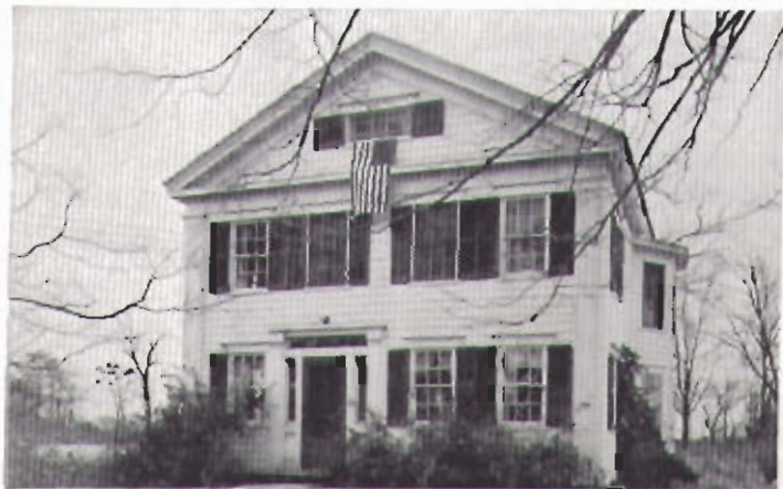
Radiant Heating replaced hot air heating in this house.
