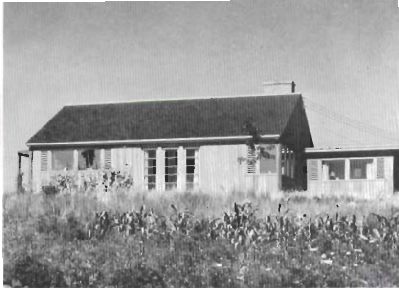
The Architect selected copper tube for Radiant Heating his home built in 1941. Despite the full exposure and large glass areas, it was heated at a very low cost.
