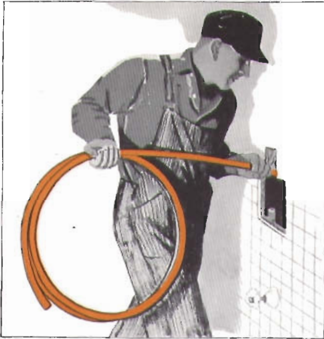
In the old days, walls and floors had to be torn open, but now with Chase flexible copper tube the plumber can snake it down through a small opening in the wall.
