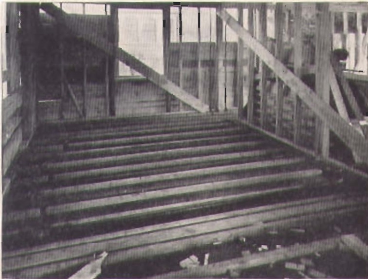
Setting floor joists on the concrete makes it easy to install ordinary wood floors above wrought iron radiant heating coils.
