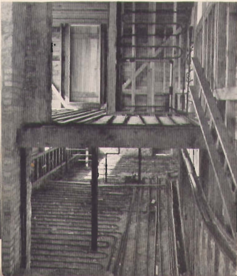
Setting floor joists on the concrete makes it easy to install ordinary wood floors above wrought iron radiant heating coils.
