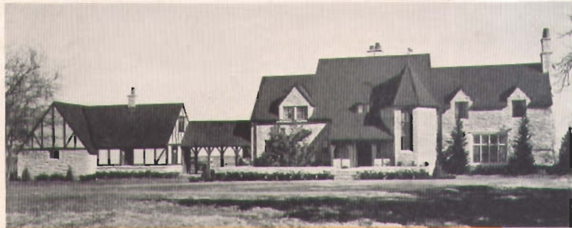
Mr. & Mrs. R. L. Hoover, Oklahoma City, Oklahoma. W. N. Eaton, architect. (Radiant heat in flower-sun room and hall.)
