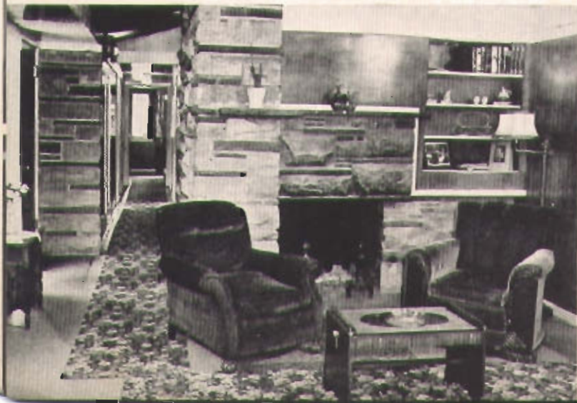
Rough stone used for the fireplace, chimney, and a portion of the outer wall, gives an unusual effect. Wrought iron radiant heating coils are buried in the floor.
