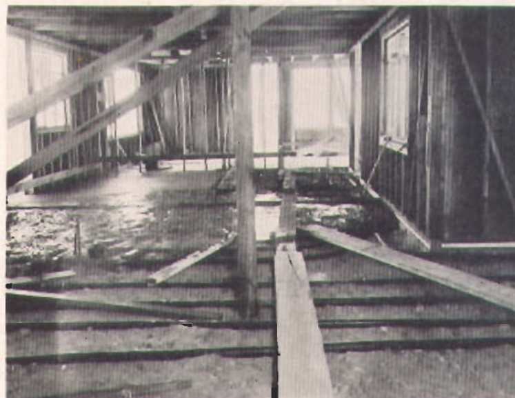
As more people get used to the idea of concrete floors, this method becomes increasingly popular. Such floors can be very attractive, and in a house with radiant heat they are entirely comfortable.
