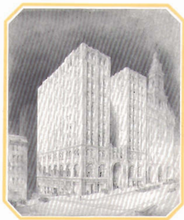
National Savings Bank, Albany, N. Y.
