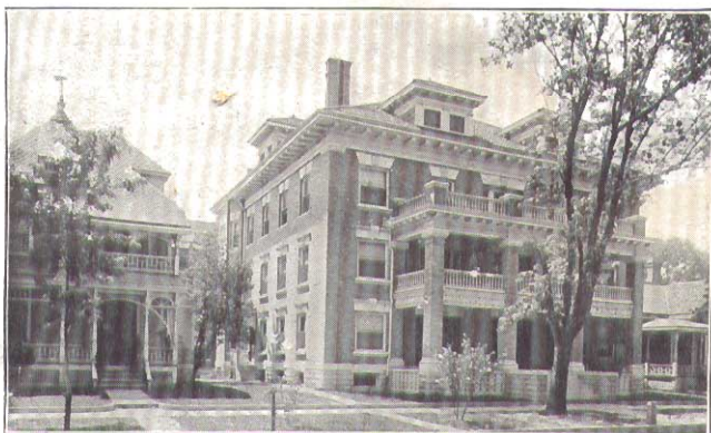
Barnes Apartment Bldg., Wichita, Kans.
