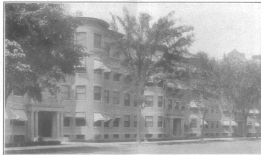
Section of a row of buildings on Beacon Street, Brookline, Mass., owned by C. A. Newhall Heated by six boilers equipped with our apparatus
