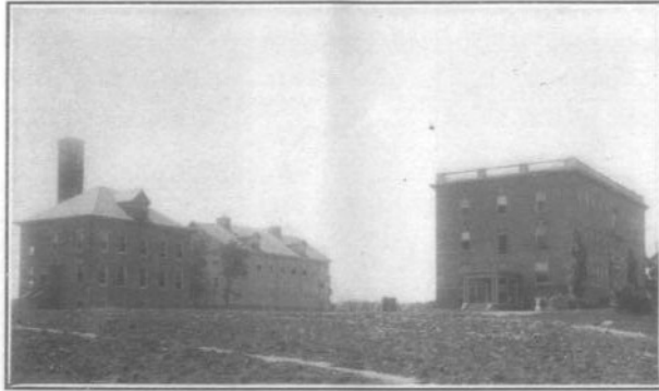
Boston School for the Deaf, Randolph, Mass. Heated by a central plant with mains carrying vapor over 100 feet under ground
