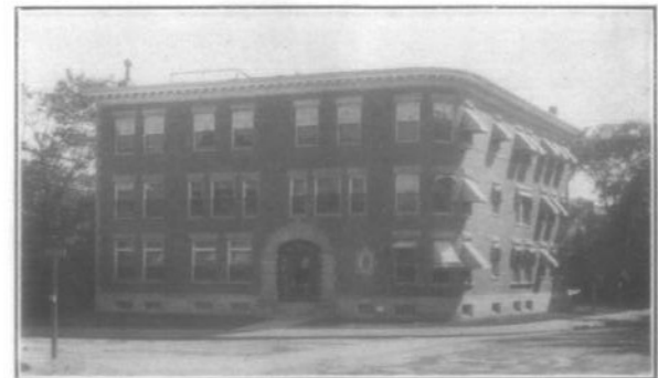
The Gorham, Gorham Street, Brookline, Mass. Heated by 41 radiators and 1,760 feet of radiation
