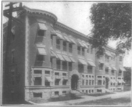
The Lincoln Terrace, Park Street, Brookline, Mass. Heated by 63 radiators and 2,630 feet of radiation
