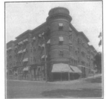
Apartment Building of A. Grosser, M. D. Warren and Copeland Streets Roxbury, Mass.
