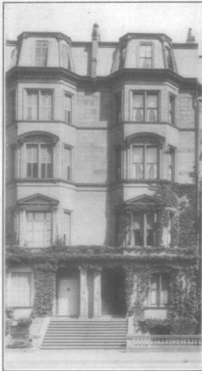
Residence of R. D. Sears Beacon Street, Boston, Mass.
