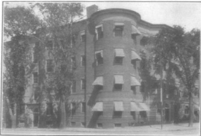
The Ambleside, Park and Washington Streets, Brookline, Mass. Heated by 56 radiators and 2,340 feet of radiation
