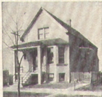
A No. 218 IDEAL Boiler and 270 ft. of 38-inch AMERICAN Radiators, costing the owner $135, were used to Hot-Water heat this cottage.
