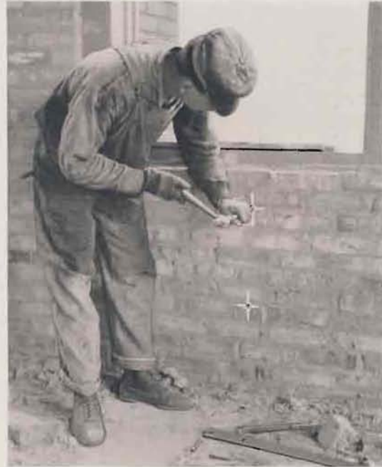
Fig. A. Chalking location of Arco Adjustable Wall Bracket, and drilling bolt-holes.
