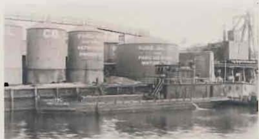
Oil Barge No. 5 of Pure Oil Co., New York, equipped with AMERICAN PEERLESS Wall Radiators. Their use herein is an aid to "Safety First" heating.
