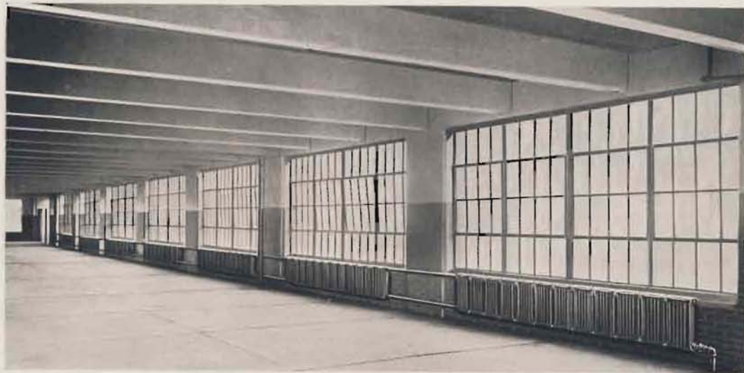
Typical floor of Hyatt Roller Bearing Company's factory at Harrison, N. J., showing 756 square feet of AMERICAN PEERLESS Wall Radiators in single run of seven units of 12 sections each—with one supply and one return connection—operating under vacuum system and with an initial pressure of 1\frac{1}{2} pounds.
