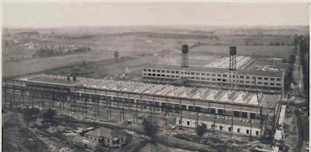
J. I. Case Threshing Machine Co. Works, at South Racine, Wis., are equipped with AMERICAN PEERLESS Wall Radiators, which are cleverly distributed to occupy a minimum of the valuable floor space.
