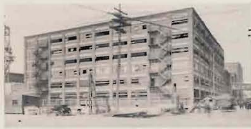
Hyatt Roller Bearing Co., Harrison, N. J. Heated with AMERICAN PEERLESS Wall Radiators on Vacuum Heating System throughout.
