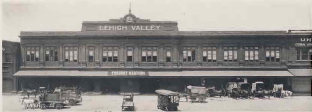
Lehigh Valley R. R. Terminal, Pier 8, North River, New York, is equipped with AMERICAN PEERLESS Wall Radiators, which stand up under all the rough conditions implied in freight transfers from both land and water.
