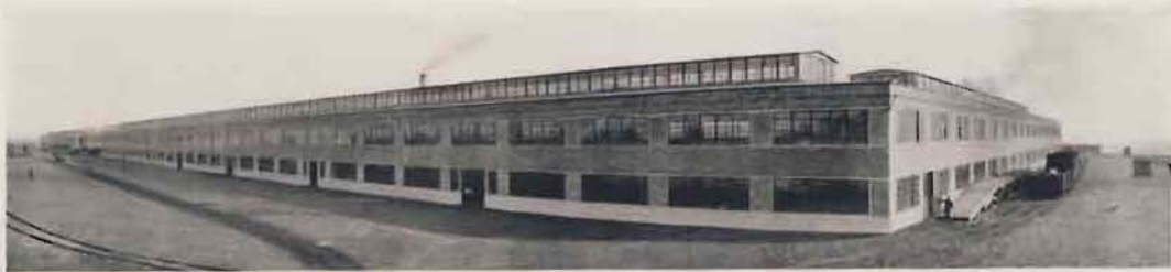
This far-stretching plant of the Eddystone Ammunition Corporation, at Eddystone, Pa., is equipped with many thousands of square feet of AMERICAN PEERLESS Wall Radiators, and offers exceptional proof of the easy-erection and space-saving qualities of this form of modern heating surfaces.
