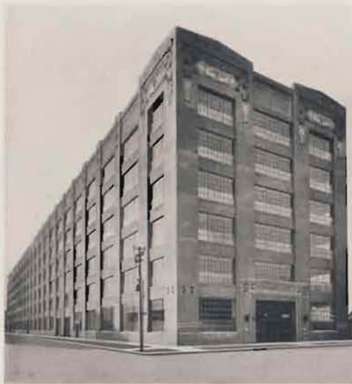
Excelsior Motor Mfg. Supply Co., Chicago. Main Building, 600 x 132, by six stories high. Built of reinforced concrete—no wood used in any part of the building. Heated with AMERICAN PEERLESS Wall Radiators and VENTO Hot Blast Heaters.
