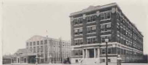
View of portion of River Works of General Electric Co., at West Lynn. Equipped with AMERICAN PEERLESS Wall Radiators.
