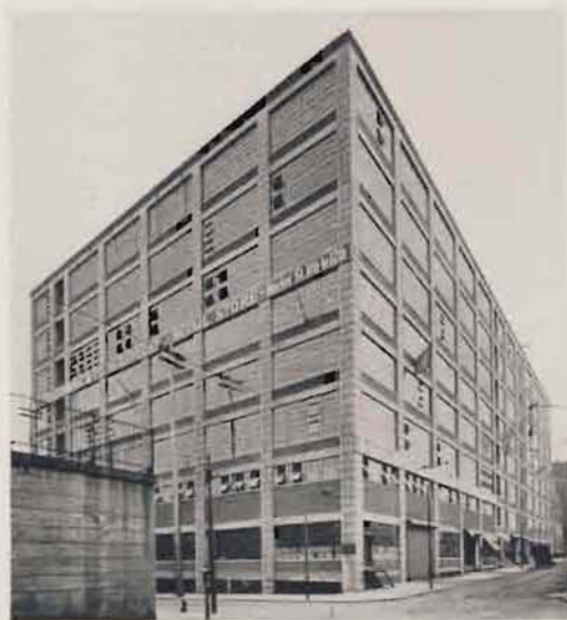
Warehouse of the great Department Store of H. Snellenburg & Co., Philadelphia, equipped with AMERICAN PEERLESS Wall Radiators.
