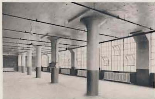
Paramount Knitting Company, Kankakee, Illinois. Equipped with AMERICAN PEERLESS Wall Radiators. Compact arrangement allows for greatest floor space, light and freedom for workers.
