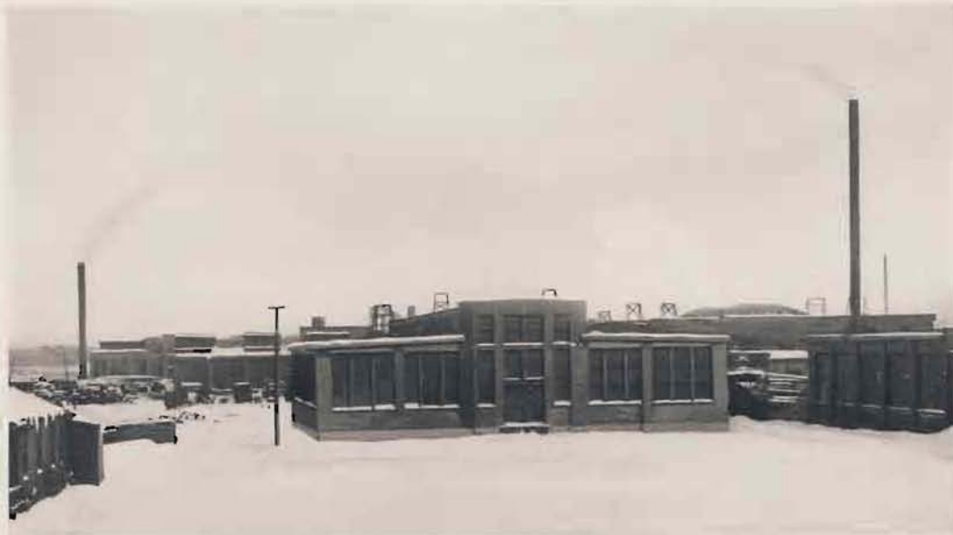
Equipment Building of American Radiator Co., at Buffalo, N. Y., where important tests of AMERICAN PEERLESS Wall Radiators were conducted in actual zero weather.
