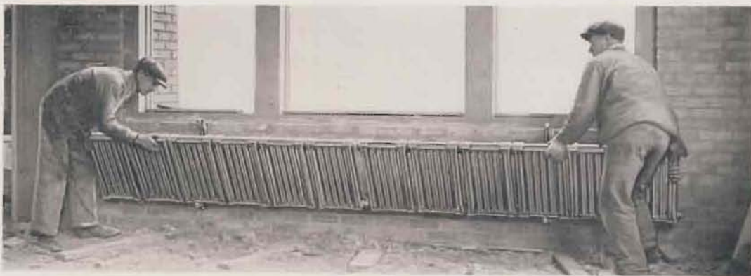
Fig. C. AMERICAN PEERLESS Wall Radiation in two stacks, connected by right- and left-hand hexagon nipples, being lifted into position on lower spools of two Arco Adjustable Wall Brackets.
