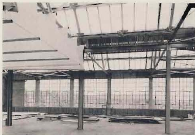
AMERICAN PEERLESS Wall Radiators below windows and along skylights in the Centaur Film Co. building—13,600 square feet of glass surface.
