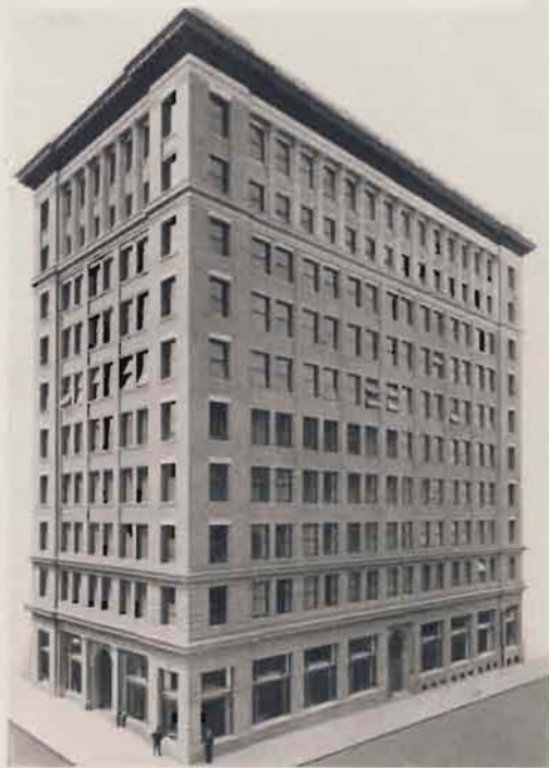
Standard Oil Company Building, San Francisco. Fuel oil is used to heat this ten-story office building. Equipped with IDEAL Sectional Boilers, AMERICAN PEERLESS Wall Radiators and VENTO Blast Heaters.
