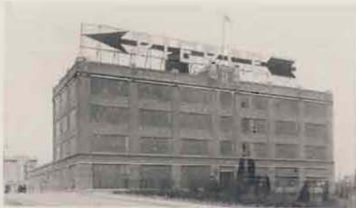
Pierce-Arrow Company Assembling Plant, Long Island City, N. Y. Heated with AMERICAN PEERLESS Wall Radiators. Forced Hot Water Circulation.
