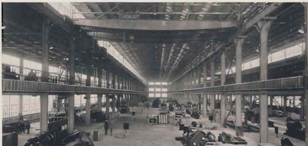
AMERICAN PEERLESS Wall Radiators in plant of The Bullard Machine Co., Bridgeport, Conn., wherein the nature of the operations requires a steady temperature of 70 degrees.
