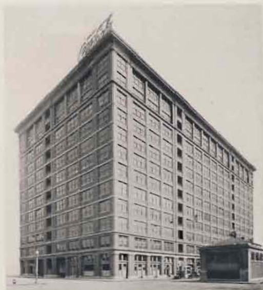
Coca-Cola Building at Baltimore, Md., equipped with AMERICAN PEERLESS Wall Radiators. For erecting view, see page 43.
