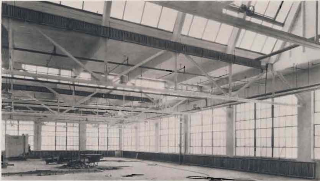
Interior view of plant of Hood Rubber Company, at Watertown, Mass., showing AMERICAN PEERLESS Wall Radiators placed in skylights and under windows.
