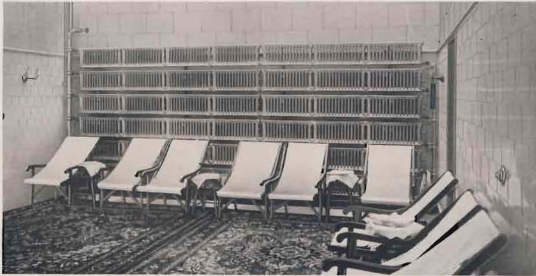
A six tier installation of AMERICAN PEERLESS Wall Radiators (in 42 sections) to maintain a high temperature in Burns' Hamman Baths, San Francisco. Compared with pipe coils (of same area) they occupy 296 square feet less wall surface, and are much more attractive in appearance.
