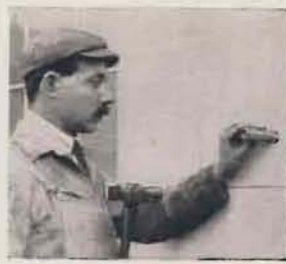
Fig. C. Inserting Shield.
