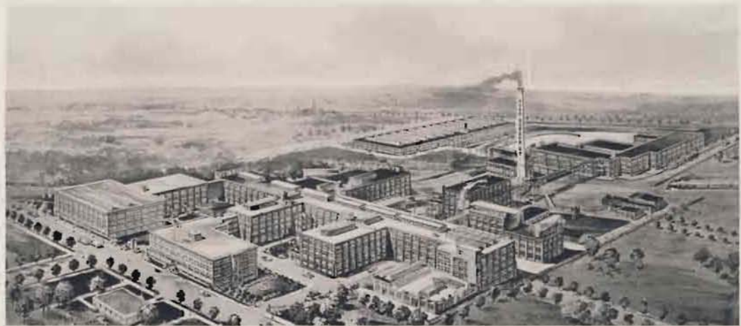
Plant of the Hood Rubber Company, Watertown, Mass., the modern buildings of which contain a large amount of AMERICAN PEERLESS Wall Radiators. These Radiators are also used in many of the modern buildings of the Goodyear Tire & Rubber Co. and other rubber manufacturing companies.
