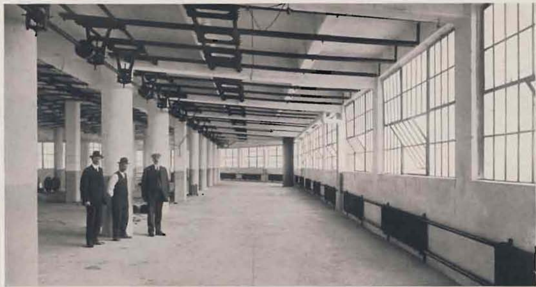
The new buildings of Thomas A. Edison, Inc., Orange, N. J., are equipped with AMERICAN PEERLESS Wall Radiators, as they filled the exacting requirements of the builder of this great scientific factory and research institution.
