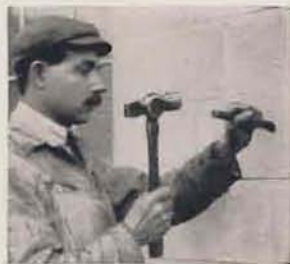
Fig. B. Drilling Hole.
