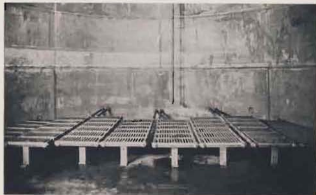
AMERICAN PEERLESS Wall Radiators used to heat creosote in a railroad tie creosoting tank.
