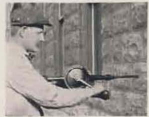
Fig. E. Using "Rapid Fire" Drill.
