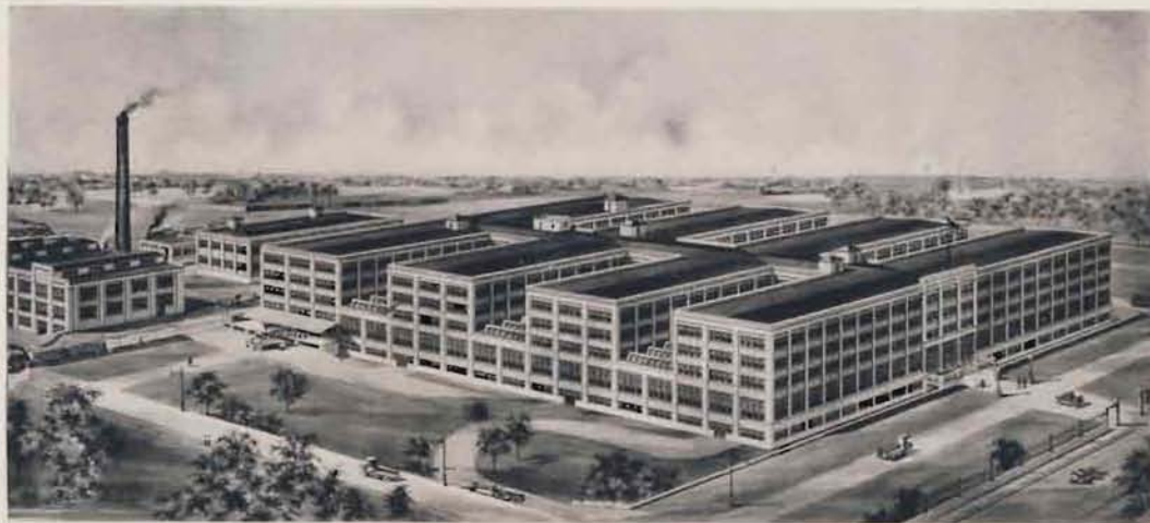
orks of the Firestone Tire and Rubber Company, Akron, Ohio. Note that more than half the wall surface is filled with windows—a tremendous area of glass surface to insure ample lighting for particular manufacturing processes. The constant chilling effects of this surface are offset by about 150,000 square feet of AMERICAN PEERLESS Wall Radiators supplied by a forced circulation of hot water—overhead delivery.
