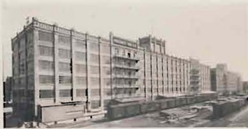
New York Dock Company Buildings, Brooklyn, N. Y. The rented warehouses lighted by large areas of glass surface are warmed by AMERICAN PEERLESS Wall Radiators.
