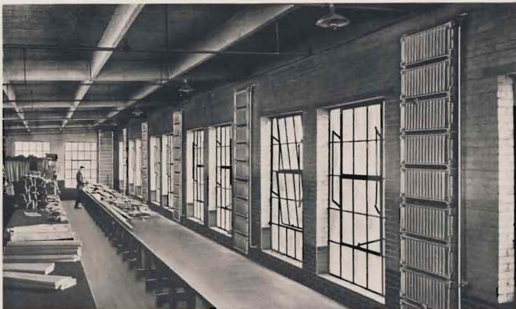
AMERICAN PEERLESS Wall Radiators in Cutting Room of Jennings Mfg. Co., at Harrisburg, Pa.
