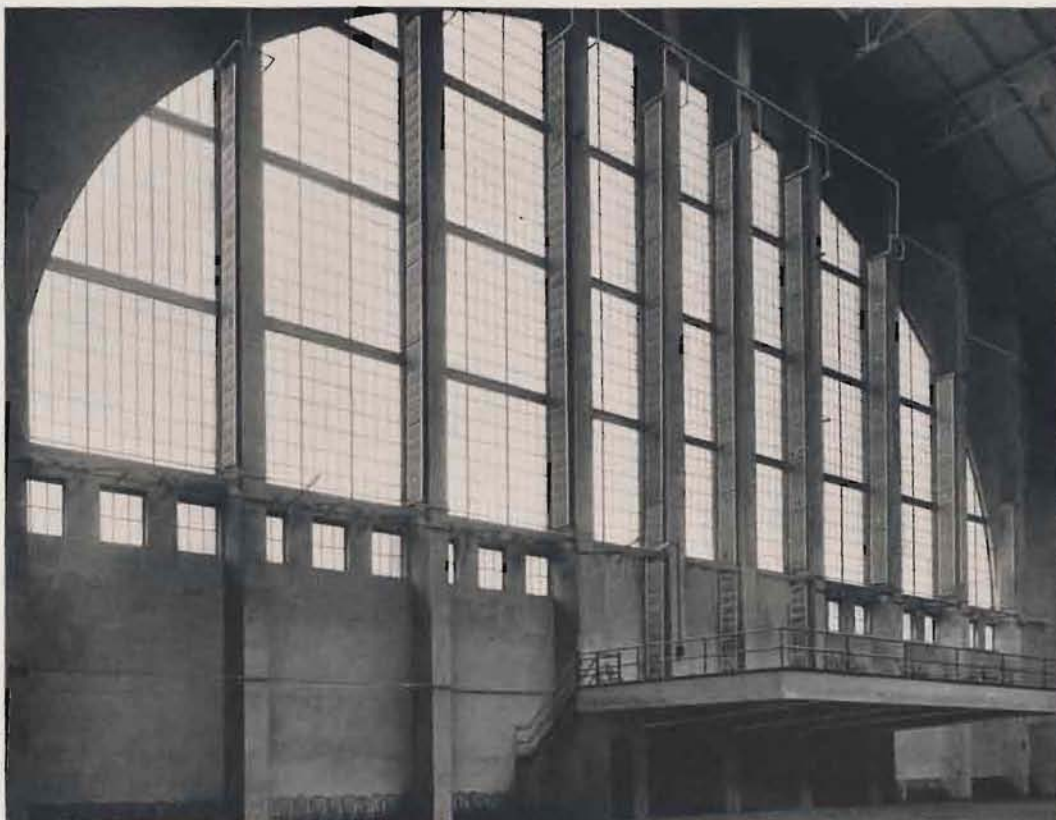
Novel treatment of a large window exposure, employing 5,886 square feet of AMERICAN PEERLESS Wall Radiators, in the Second Regiment Armory, Chicago. These long radiator columns successfully offset the cooling effect of the large glass surface without interfering with the light or accessibility of the windows.
