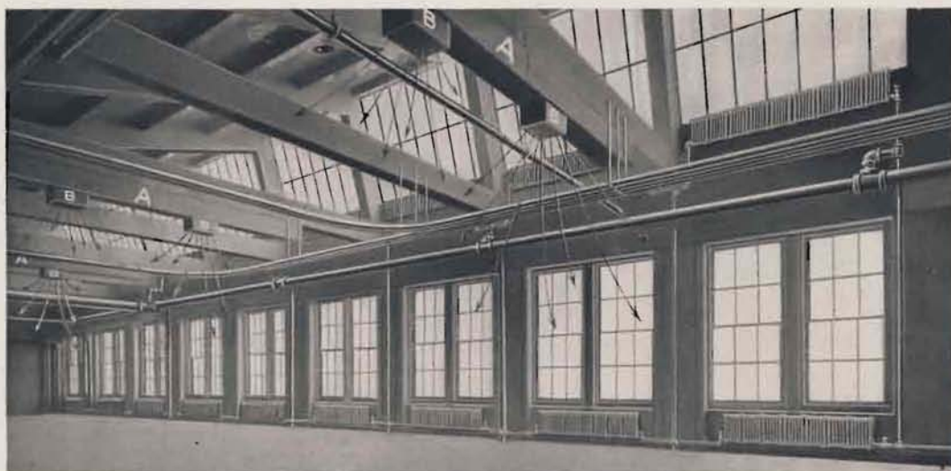
Color proving pressroom of The Curtis Publishing Company, Philadelphia, showing fresh air ducts (A) and delivery of warm air (B) from VENTO Heaters; also showing how thoroughly AMERICAN PEERLESS Wall Radiators provide heating surfaces under large side and mansard windows which insure ample light for exacting operations. A good example of combined direct and indirect heating.
