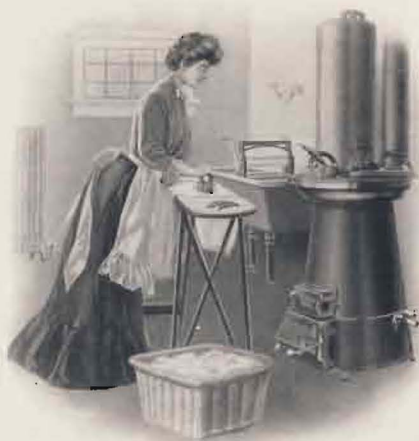
IDEAL Arco Water-Heater, also used for laundry and ironing work
