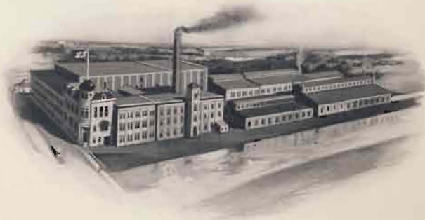
Canadian Plant, at Brantford, Ont.
