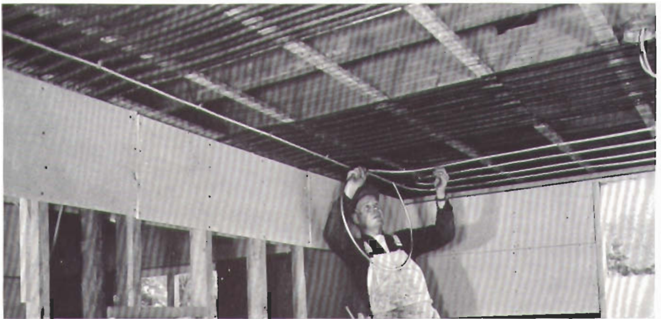
FIG. 6. "SINUOUS COILS CAN BE FORMED IN POSITION..." NOTE USE OF HELICAL BENDING SPRING.
