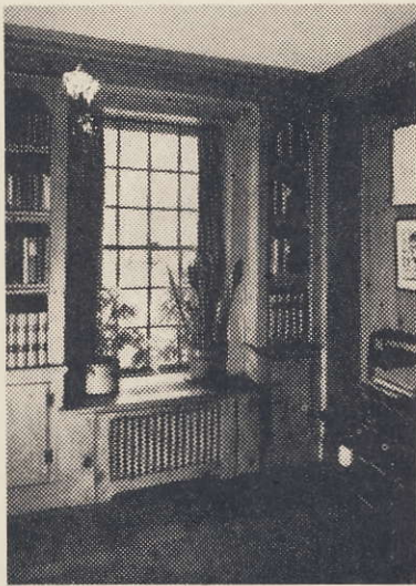
The modern slender tube, free-standing radiator may be recessed to blend with the decorations.
