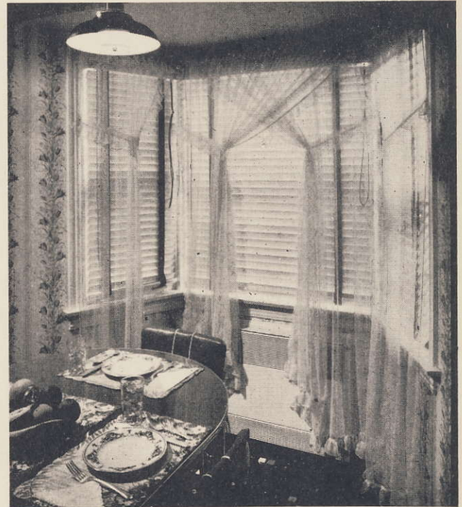
This new style radiator provides both convected and radiant heat because the front and grilles are part of the unit. Suitable for use with steam or hot water.
