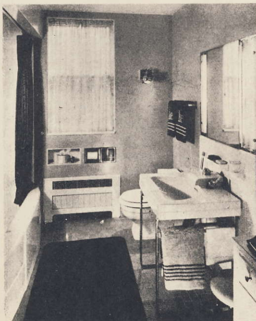
Ideal for the bathroom is the small radiant front convector, a heating unit which may be installed under the window and out of the way.
