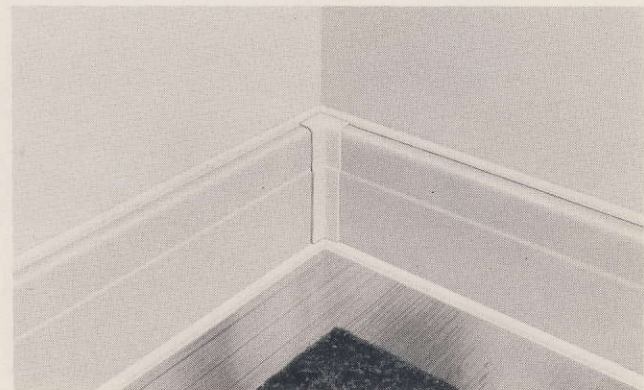
Fig. 13: Finished corner with all moldings in place.
