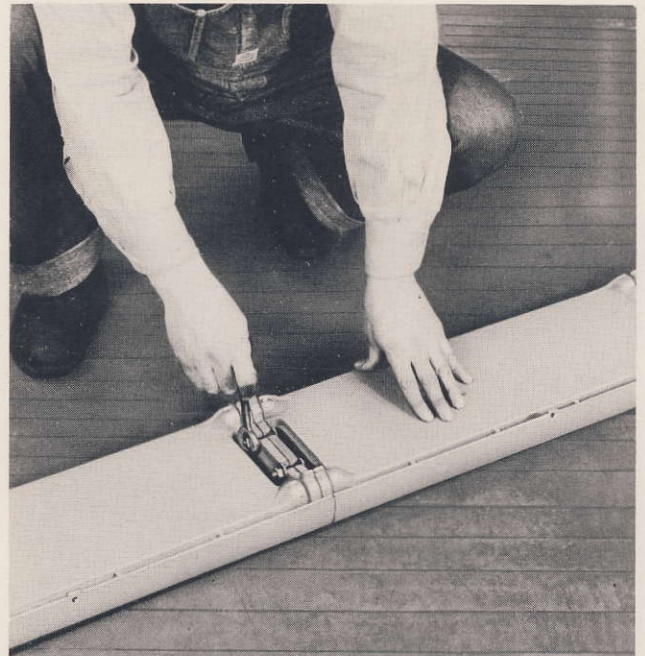
Fig. 3: Installing tie bolt between panels.
