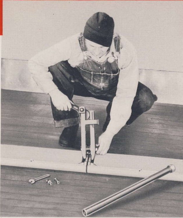
Fig. 1: Tool for assembling Radiant Baseboard Panels.
