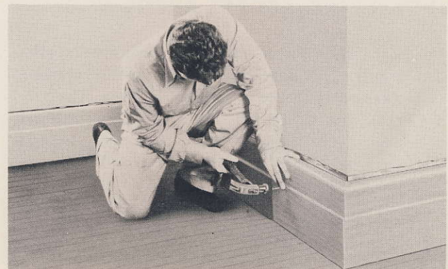
Fig. 15: Matching wood baseboard permits continuity of appearance all around the room.
