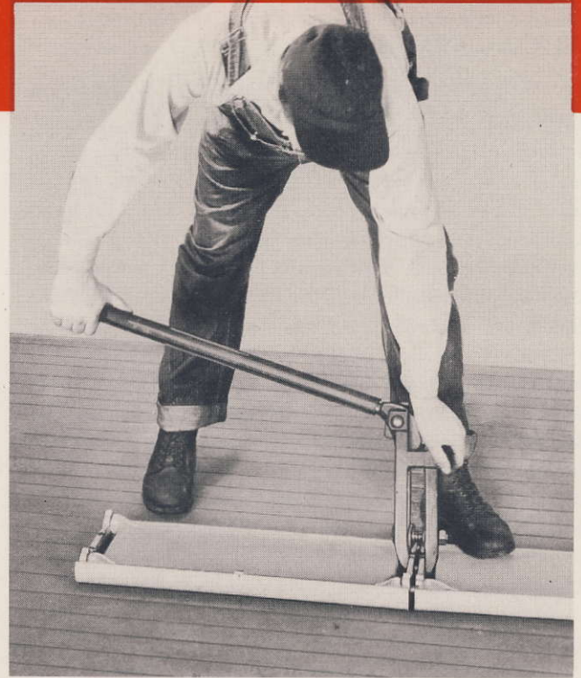
Fig. 2: Assembling Radiant Baseboard Panels.
